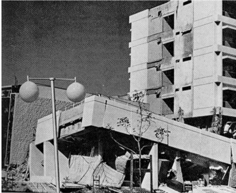
Figure 1. Collapsed Olive View Hospital
